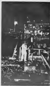
A LONELY check point in the Fire Water Pump House area where a fire security station is located.
